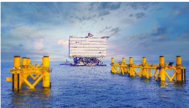
China Three Gorges Corporation (CTG) RUDONG offshore wind converter station
