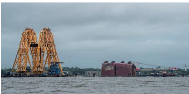
The VB-10000 began a refitting period on Sunday to prepare for the final cutting operation on the remainder of the Golden Ray wreck. Two sections remain. St. Simons Sound Incident response photo.
